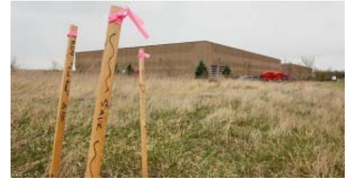
American AGCO is planning a 96,000-square-foot expansion to its existing buildings at 7800 and 7900 97th St. S. in Cottage Grove. (Staff photo: Bill Klotz)
