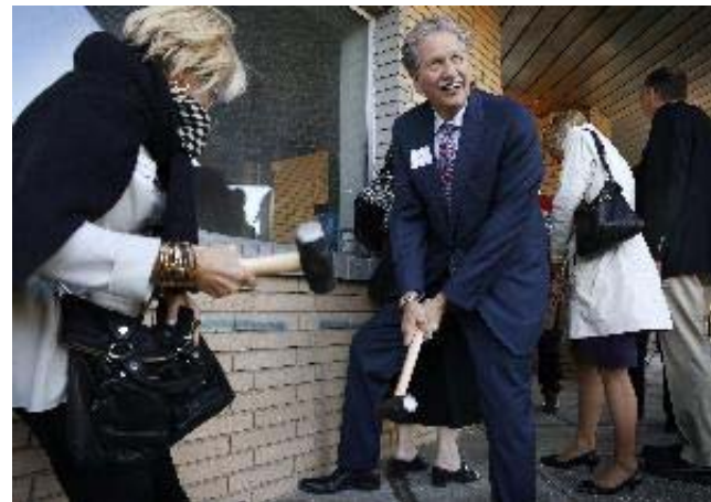
Edina Mayor James Hoyland was among those taking a swing at the Pentagon Park office park demolition party. Hillcrest Development plans a mixed-use development with at least one hotel. The project could top $500 million.
