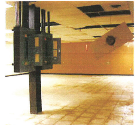
"Before" picture of the warehouse at 5121 Winnetka.
