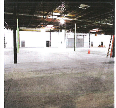
"After" shot of interior renovation.
